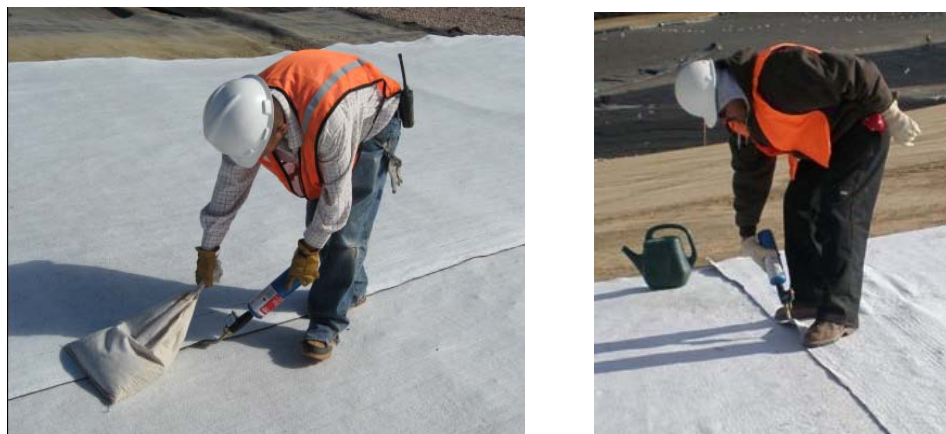
Figure 6. Installer heat-tacking GCL edge seam with a 150 mm overlap.
