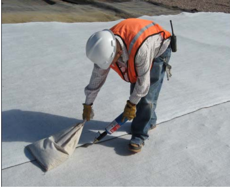
Figure 1 - Heat-tacking GCL panels with a 150 mm overlap to form a seam.
