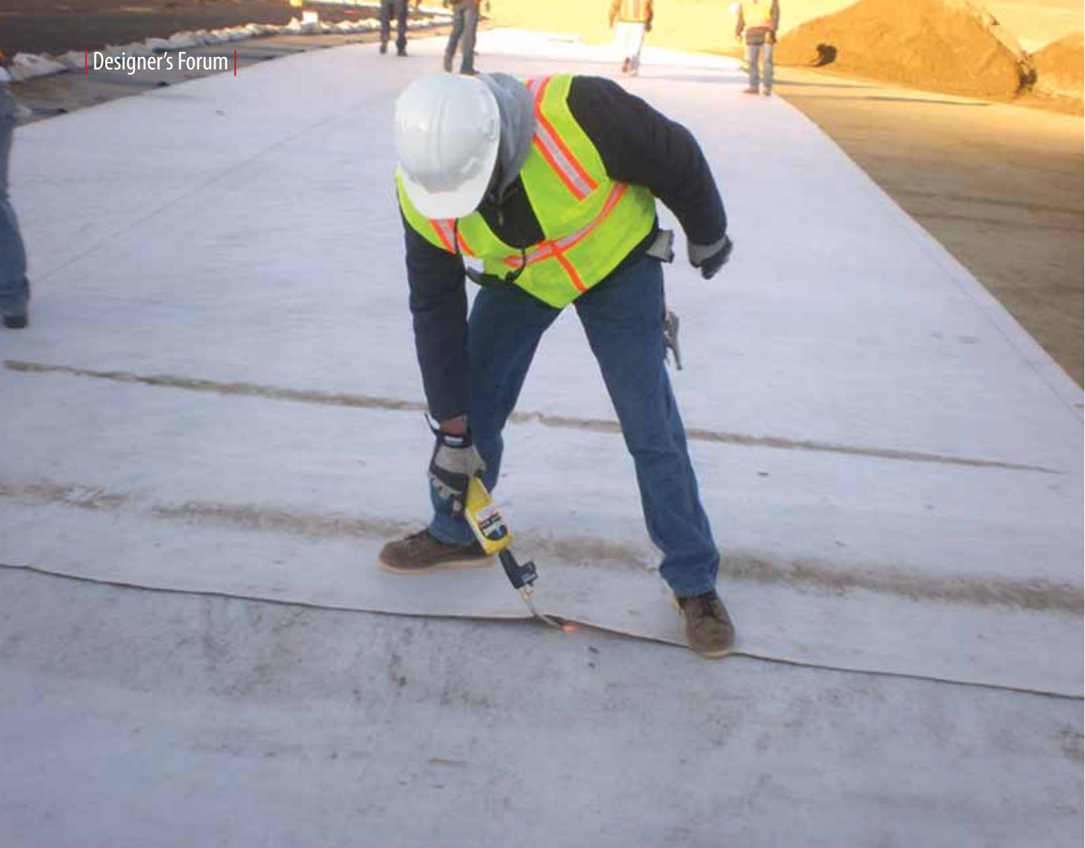
Figure 5 | Installer flame-tacking GCL butt seam.
