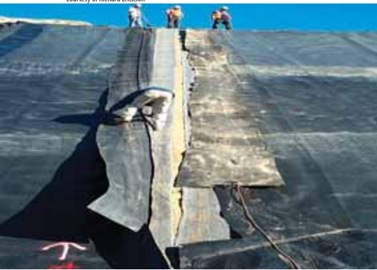
Figure 2 | GCL gap on sideslope in California.
