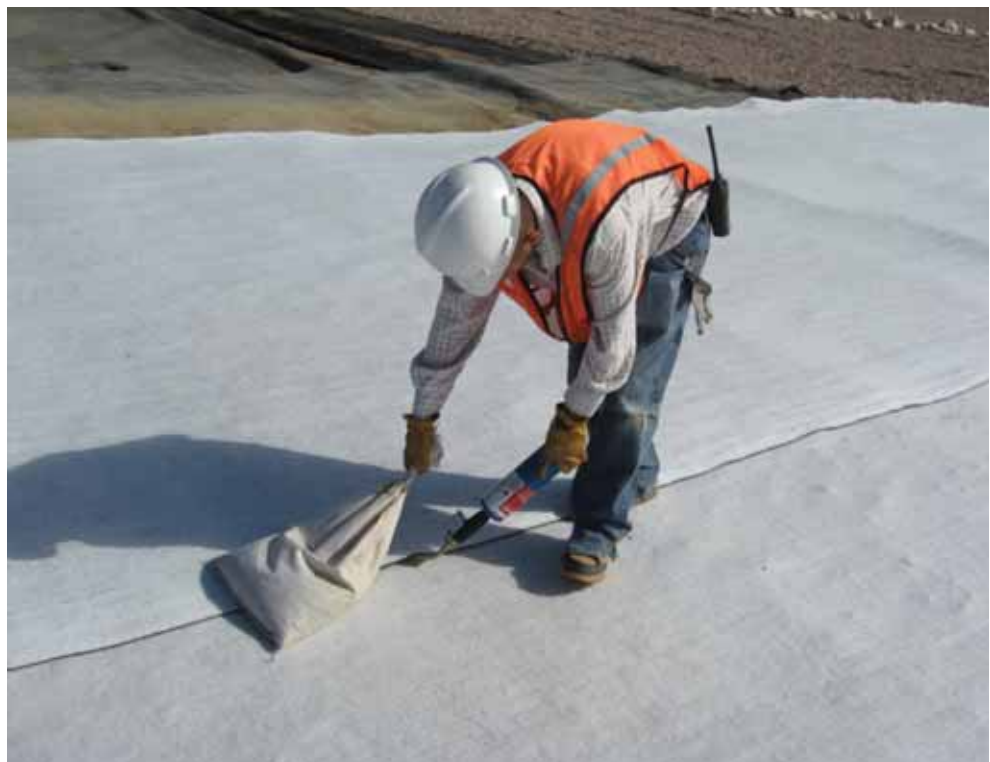
Figure 4 | Installer flame-tacking GCL edge seam having a 6-in. overlap.
