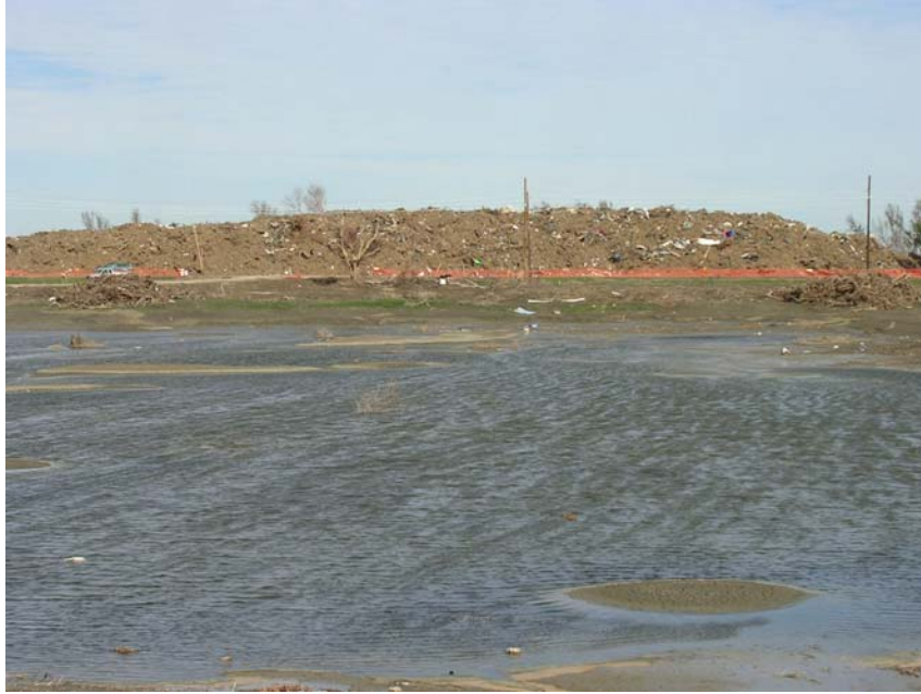
Figure 2. The Empire Pit prior to dewatering. Temporary storage and processing of waste adjacent to the borrow pit.
