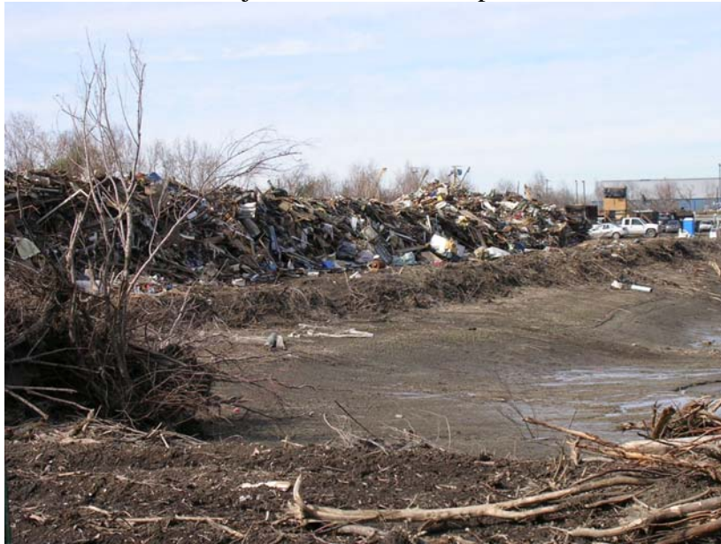
Figure 3. The Empire Pit after dewatering. Processed and staged waste adjacent to the borrow pit for final disposal.
