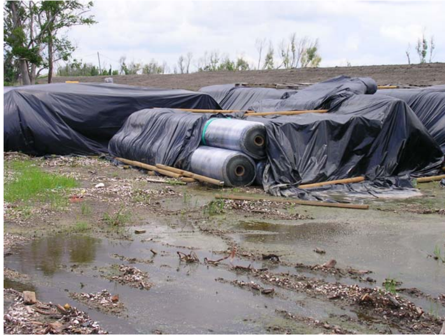
Figure 9. Storage of the GM-GCL geosynthetic material for final capping.
