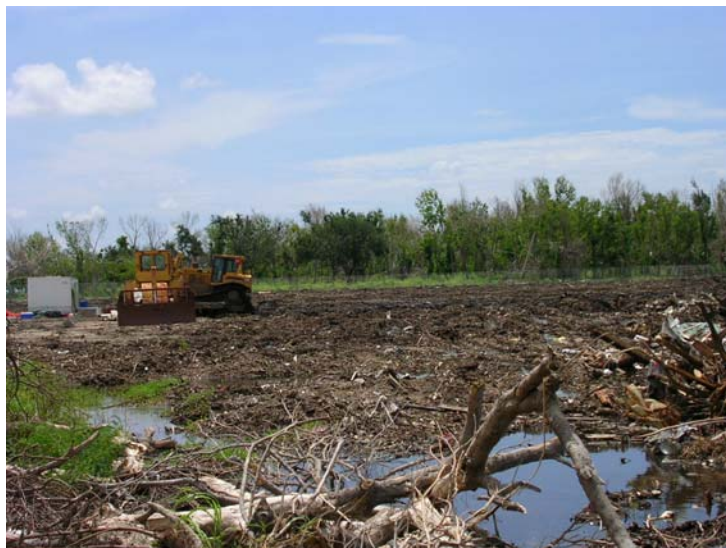
Figure 8. Waste fill approaching final grade.
