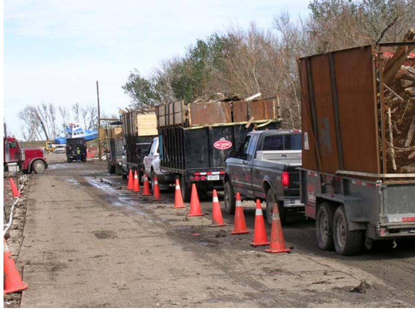
Figure 4. Incoming waste haulage and inspection.
