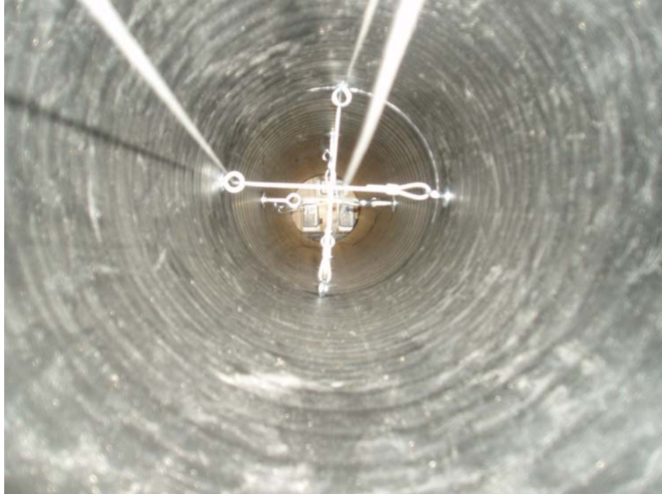
Photo 2 - Deflection Measurement System Before Test
