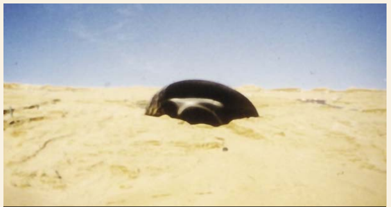
Photo 1. Geomembrane gas bubble during final cover construction.
