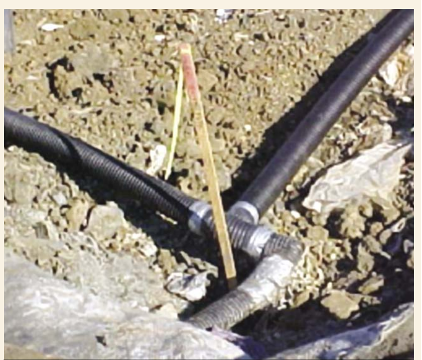
Photo 3. Vent and leachate collection seep pipes installed below geocomposite.
