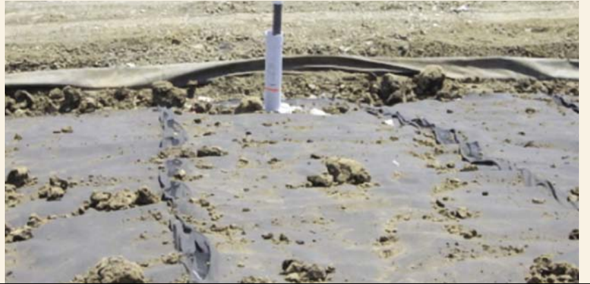
Photo 2. Geocomposite placed directly on waste interim cover—below final cover construction.
