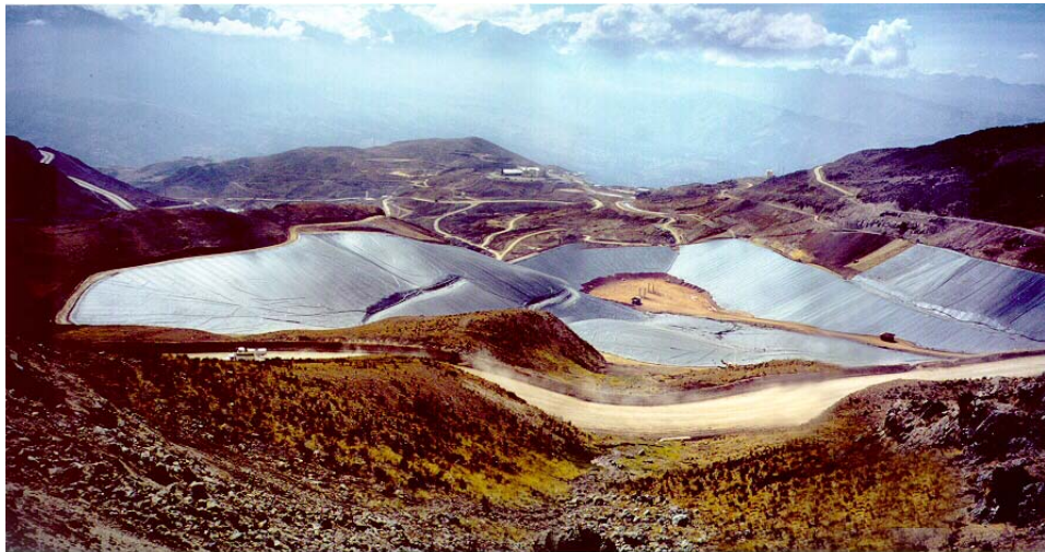
Photo note: Lined area shown is approximately 65 ha. Ultimate area will be 150 ha. Slope on right side is 1.75h:1v inter-bench angle. Commissioned in 1988.
