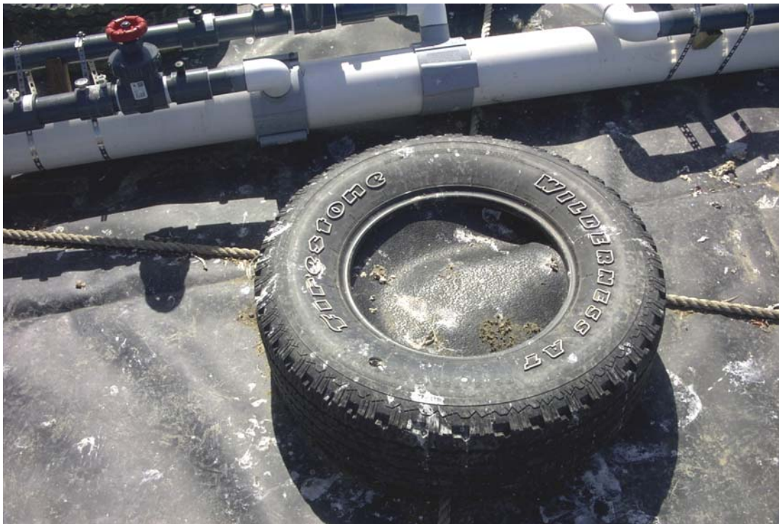
Figure 5. Photo of Tire Protection Over Sandbag.
