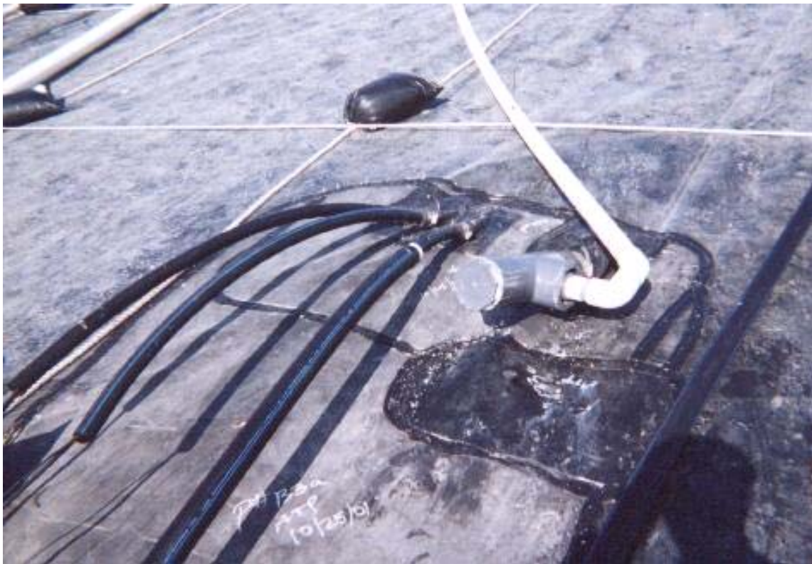
Figure 4. Photo of Pipe Penetration Group.
