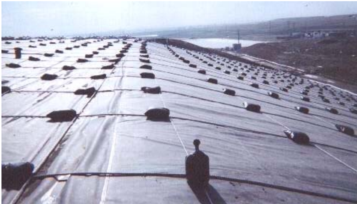
Figure 1. Completed Exposed Geomembrane Cover System from Top Crest of Slope.
