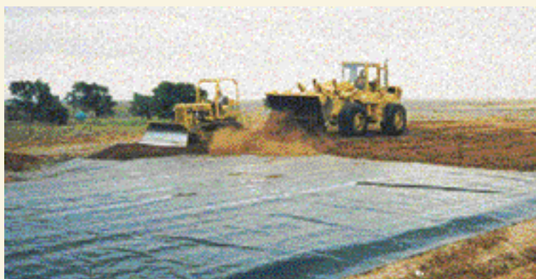
Photo 4: Soil cover placement over a GCL.
