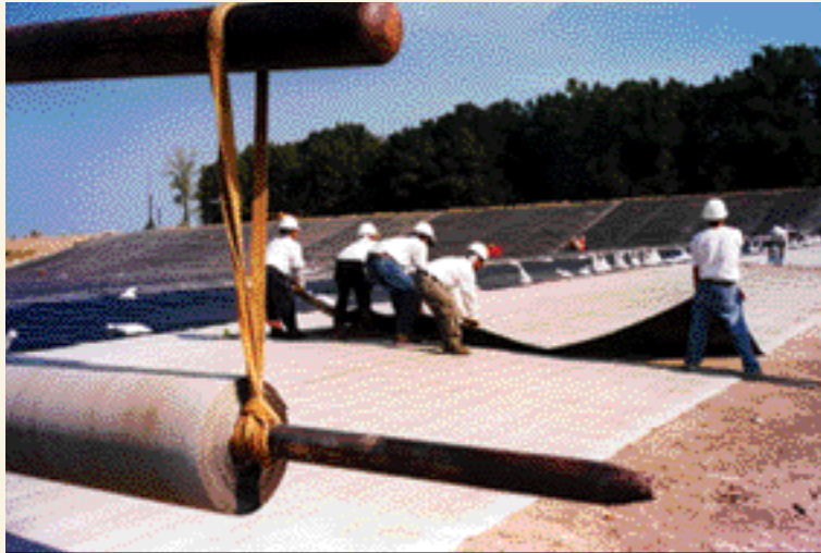
Photo 3: Final manual alignment of a deployed GCL.
