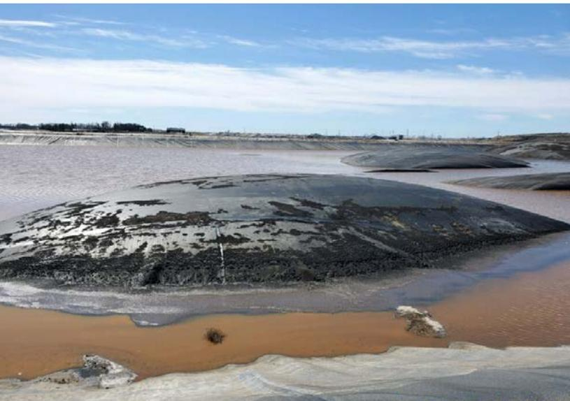
**FIGURE 1** Bubbles in pond with 60-mil (1.5-mm) HDPE geomembrane on verge of bursting.
